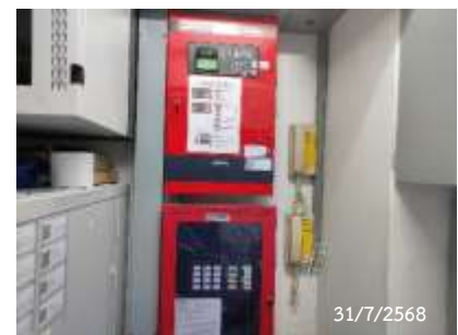
Fire Alarm Control Panel
