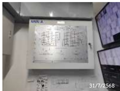
Graphic Annunciator Fire Alarm System
