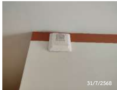
Fire Alarm Horn Strobe
